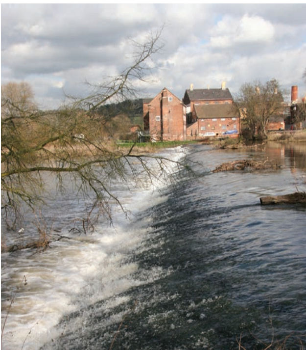
Engineered river channel at Burton Mill (Nick Mott)
