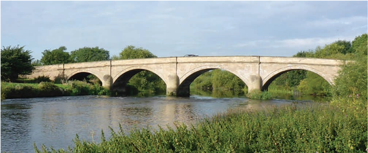
The medieval Swarkestone Bridge, Derbyshire ( ArcHeritage, 2017 )
